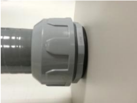
Figure 6. Gasket and Conduit installation
