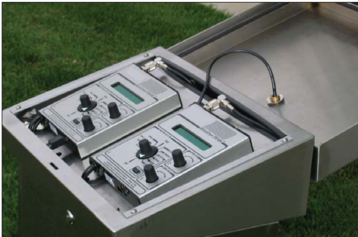
The dedicated commercially landscaped, metered sites with an ET controller showed average savings of 472 gpd.
